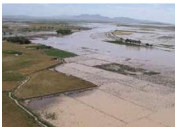
Large areas of agricultural land flooded in Sharana, Paktika Province. Flood walls will prevent such damages from happening in the future.
