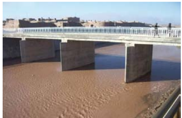
Qarya Jaya Bridge reinforced and paved on by PRT Herat.
