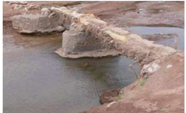
Qarya Jaya Bridge before its reconstruction.
