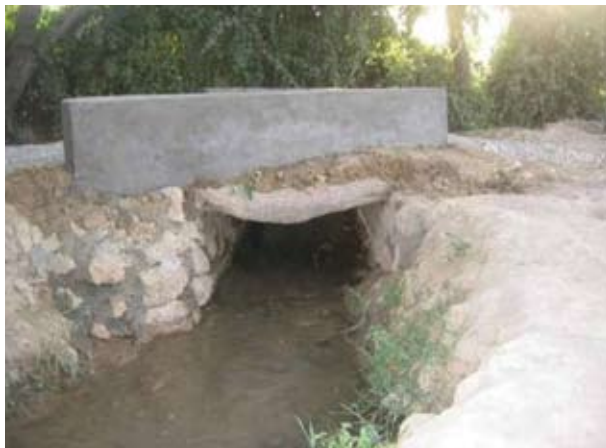
Canal bridge in Chora district repaired by PRT Tarin Kowt.
